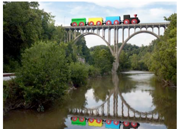
Busy Little Engine travels through many interesting landscapes on his adventures. Here, Busy Little Engine crosses a very tall bridge.
